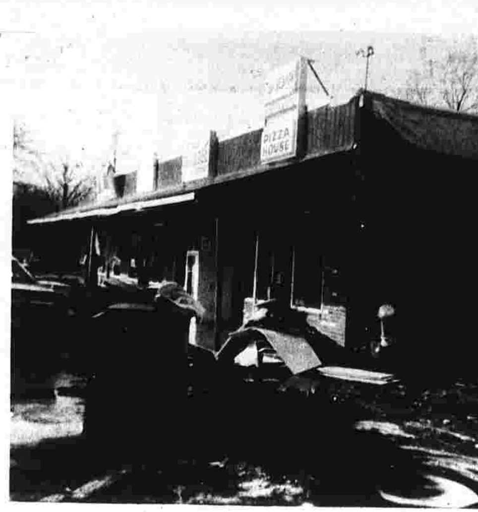
The Hebron Pizza House sustained heavy damage in Monday's storm when wind blew away a section of the roof. (Herald photo by Dallaire)
